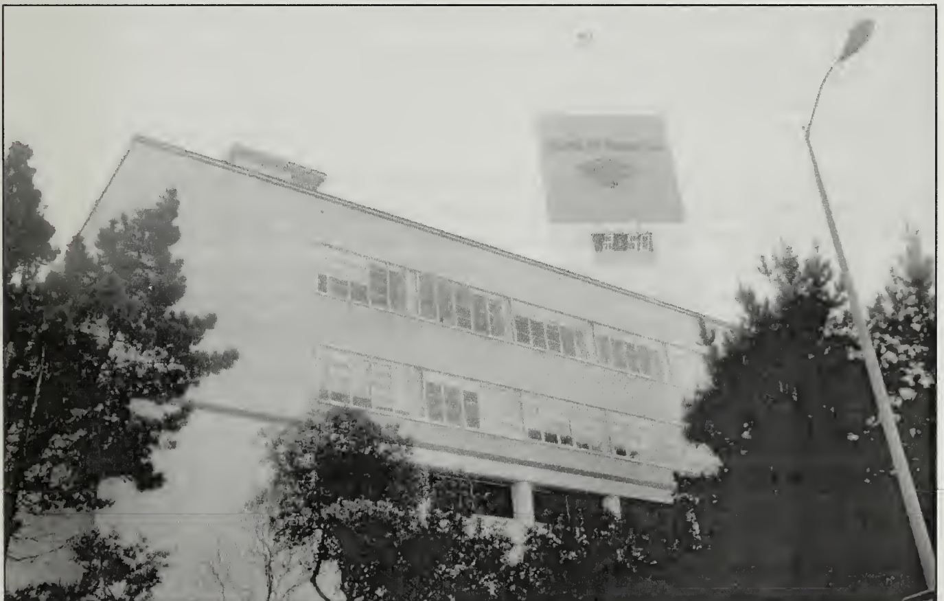
Figure 43 - Office Building, East Facade (Harrison Street Off-Ramp)
